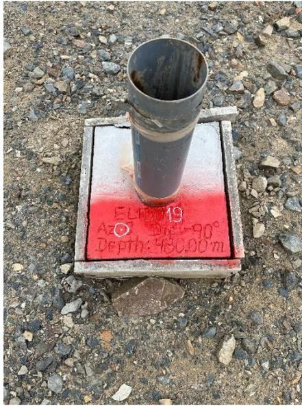
**Figure 12-15: Typical drill hole collar monument from Element 29's 2021 drilling campaign.** Source: S. Park (2022).
